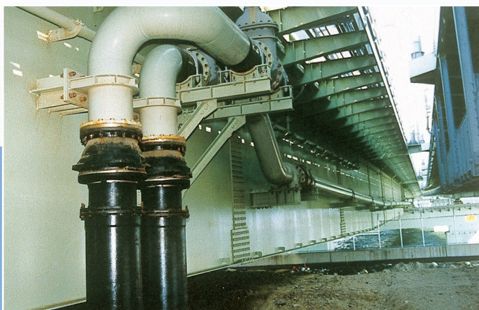
GEOFLEX® single ball joint DN 400 Overhead traverse in pipe gallery
